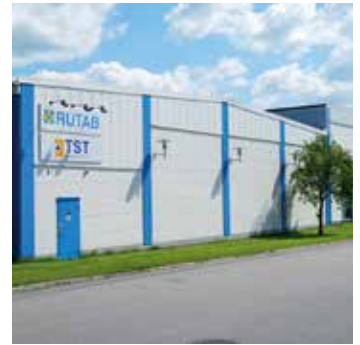
Warehouse - and production facility in Nässjö, Sweden
