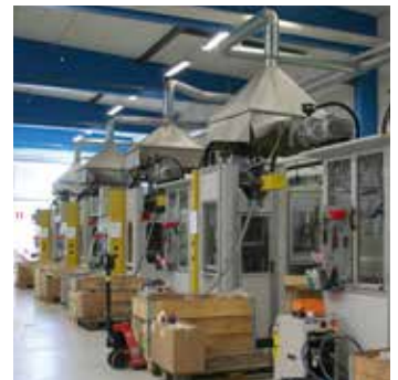
Production facility in Nässjö, Sweden
